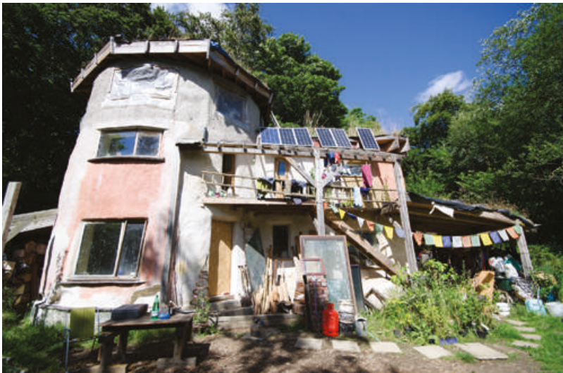
Figure 4.3 Almost complete straw bale and turf-roofed house at Green Hills (© Jenny Pickerill)
