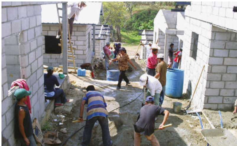
Figure 13.7 The FUCVAM self-build co-operative housing initiative in Uruguay (Photo credit: BSHF)
