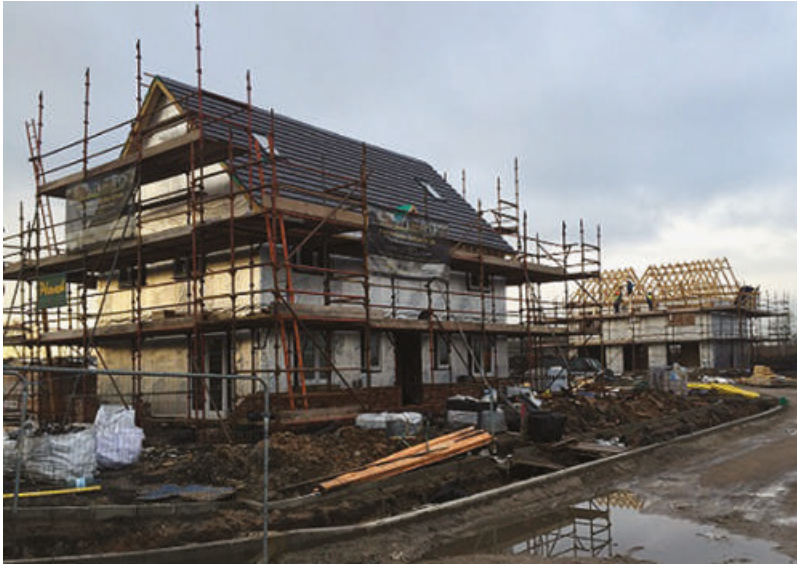
Figure 13.10 The homes on the first Potton site near St Helens are now coming out of the ground (© Buildstore)
