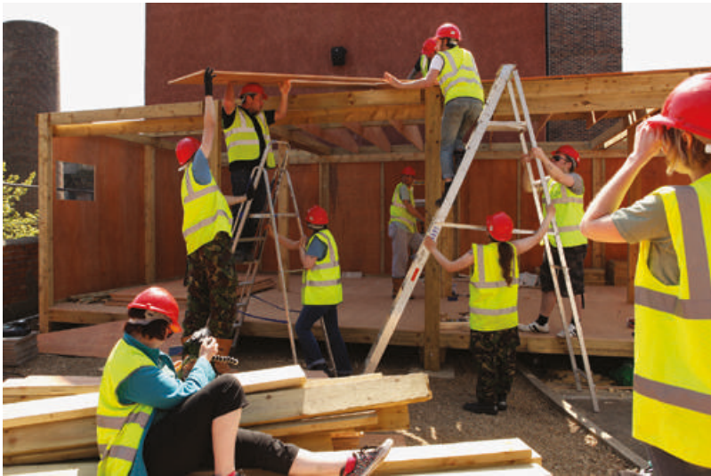
Figure 6.5 The site build (Photo credit: John Hipkin)
