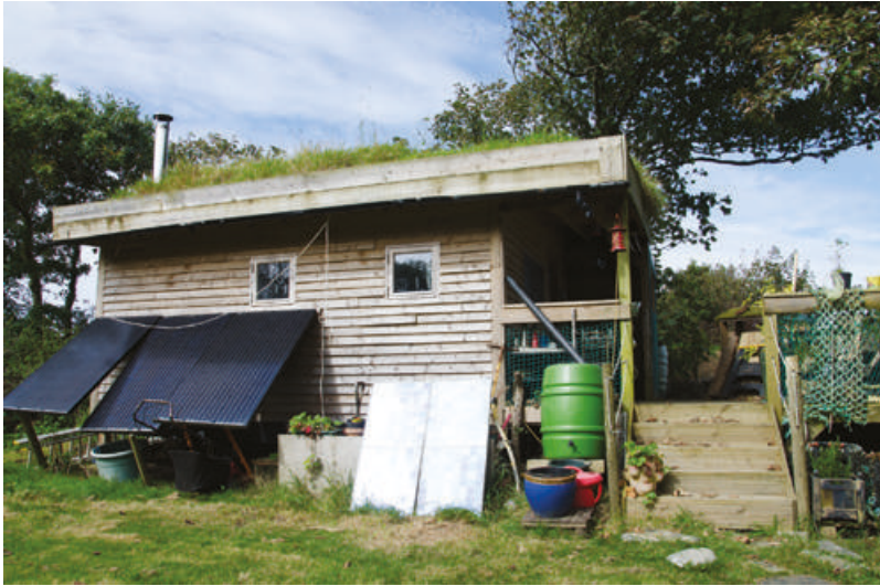
Figure 4.6 A ‘tiny home’ at Trelay community, Cornwall (© Jenny Pickerill)
